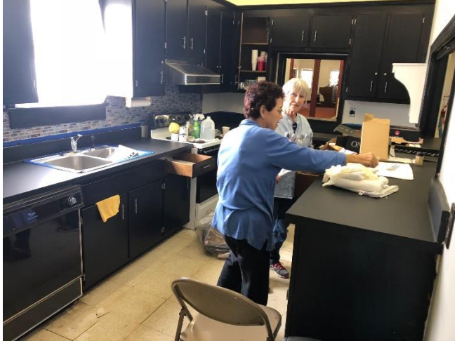
Renovating the Kitchen at St Timothy's Chapel
